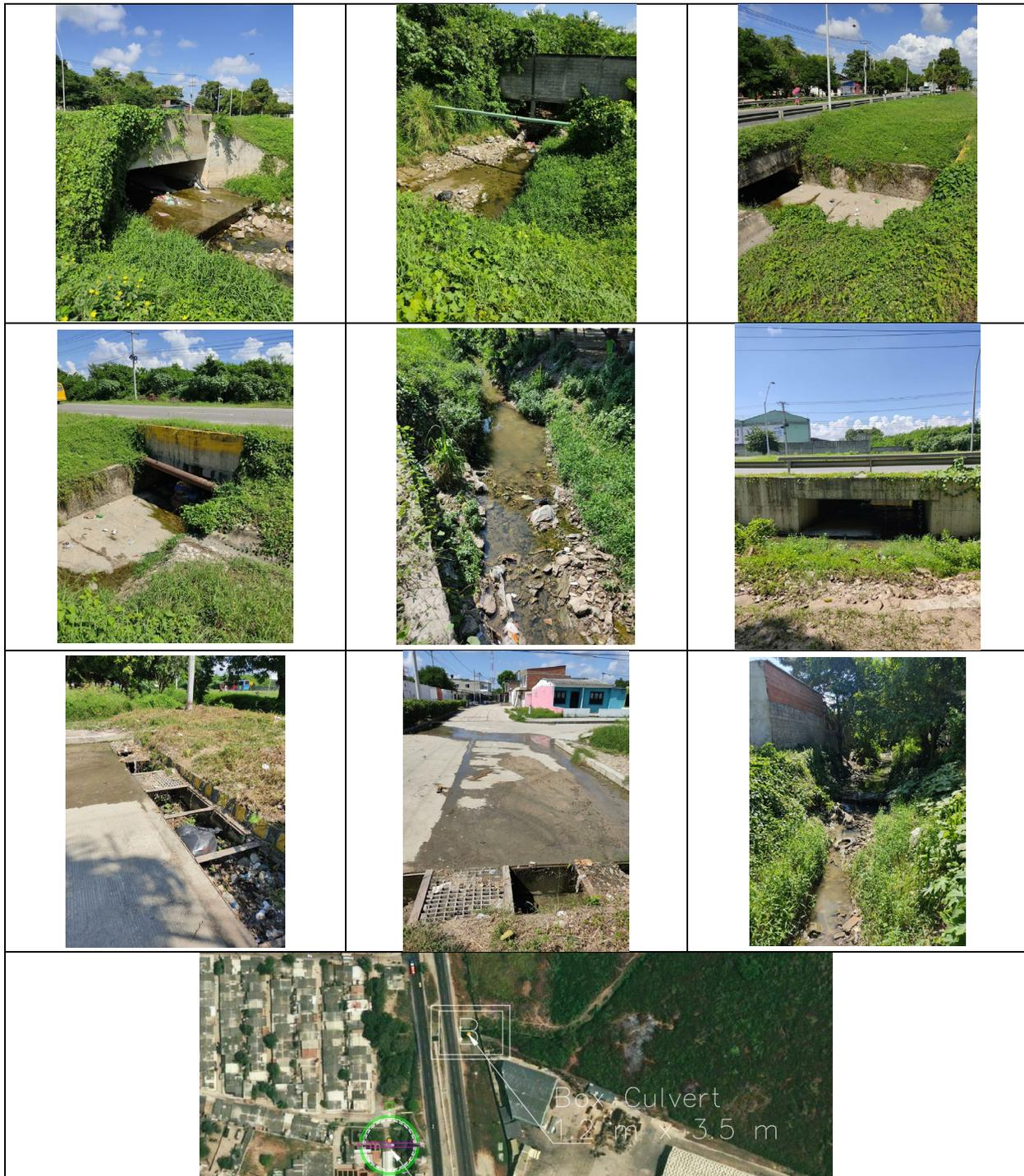
**Figura 117. Box Culvert “1.2 x 3.5 m”.**
